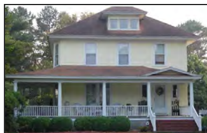
Source: Large wrap around - note the gable roof line over the porch entry
