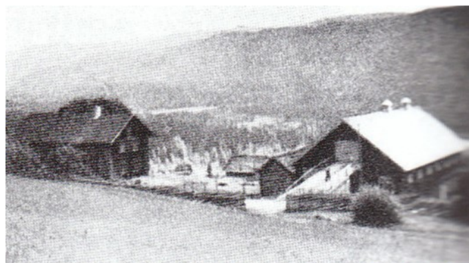
Nedre Ulland as seen from the Saksumdal Road. Note the barn to the right with a ramp going to the upper floor. Hay could be loaded directly to that floor and thrown down to the animals below. ( Husmanns-plasser i Fåberg , vol. 1, Fåberg Historielag, 2005.)
